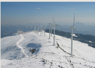
Wind turbines in cold climates
